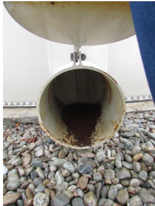
Overflow has flap, unknown if screened
