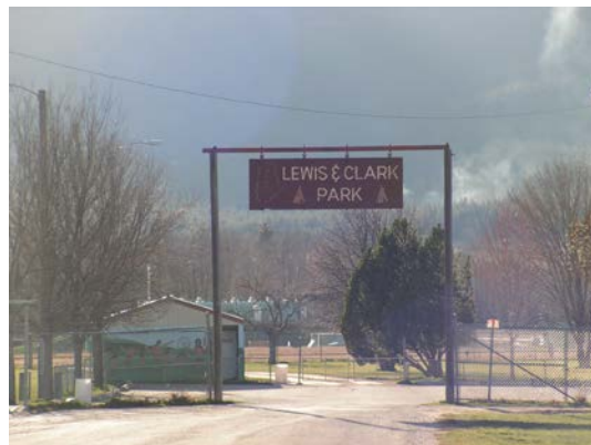
Figure II-1. The Stevensville WWTP is located directly adjacent to Lewis & Clark Park and the Town's public swimming pool.
