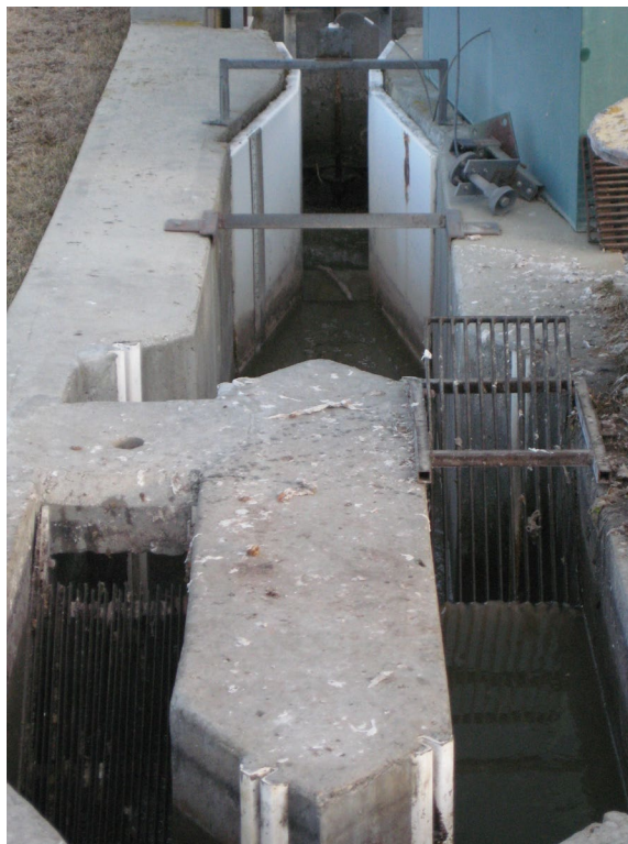
Figure II-1 Photograph of influent screen and Parshall flume showing the modifications to the screen on the left.
