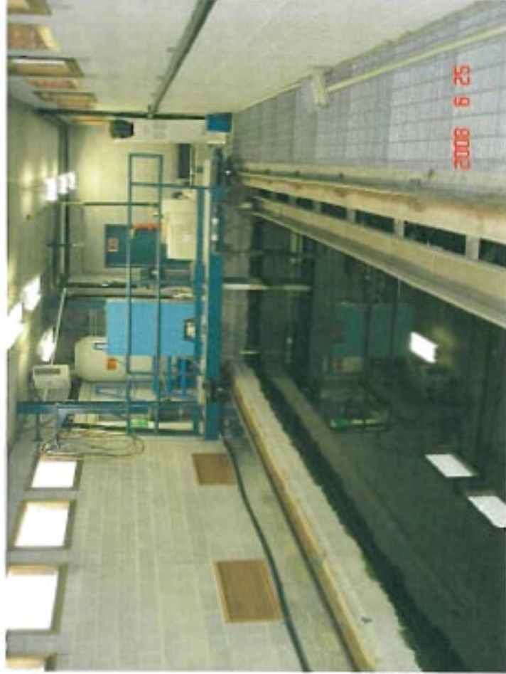
Top left: Surface water inlet from Swamp Creek and Mill Creek sources (TP001). Excess water flows over a wall at the far end of the entry basin and goes to storm drain. Coagulant (alum) is added and flows through settling basin. Chlorine injection is available at this point, but is not used.
