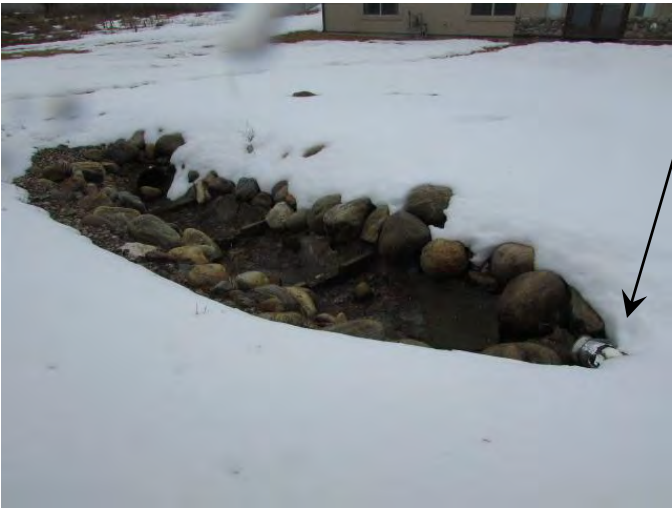
Line from Lakos unit to waste outside, with screened termination
