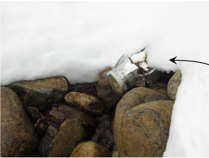
Line from Lakos unit to waste outside, with screened termination
