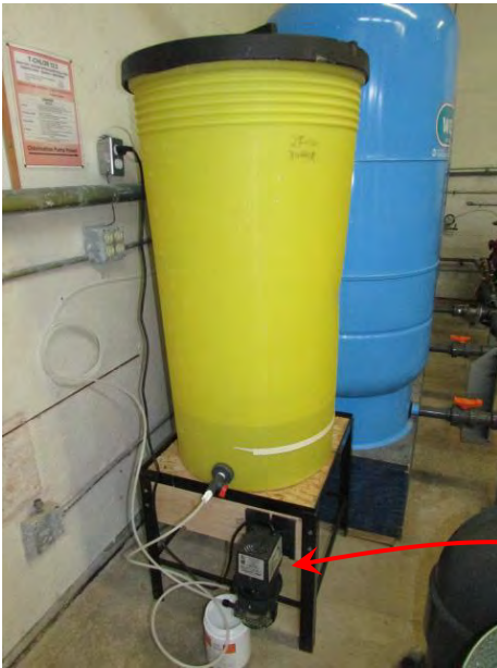
TP for Wells (TPO01) step 2: Disinfection with sodium hypochlorite
