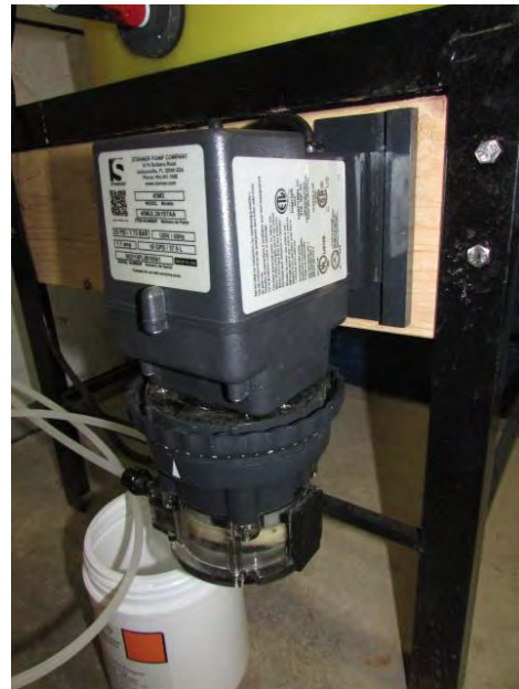
Chemical pump - Stenner peristaltic pump
